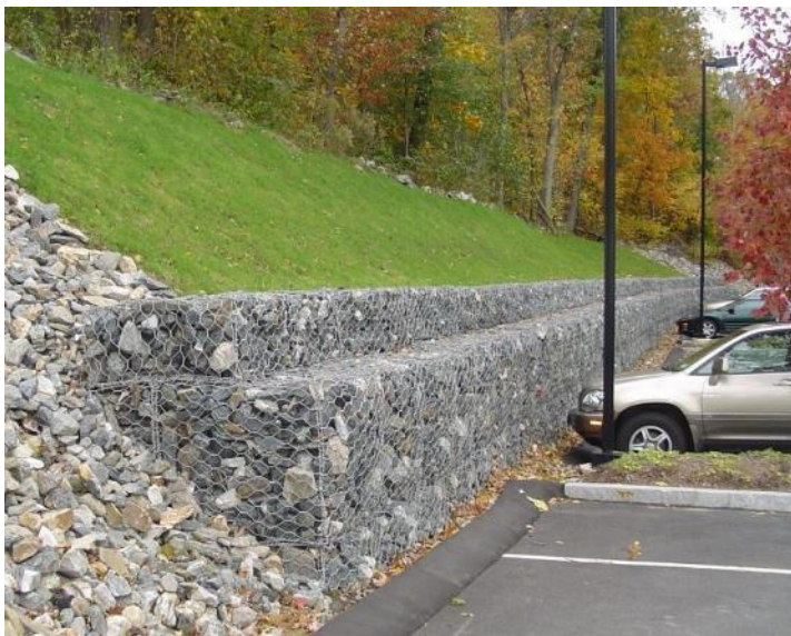
Figure 31 – Typical Gabion Wall
