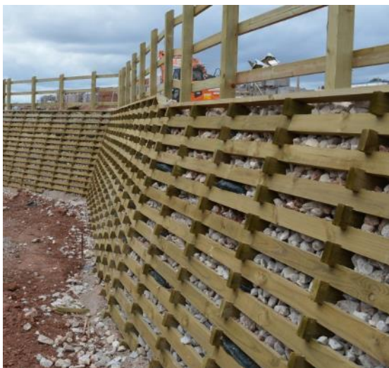
Figure 30 – Typical Permicrib Wall under construction
